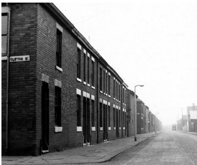
Old workers housing of Miles Platting
